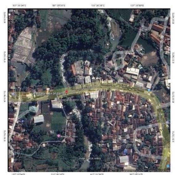
Figure 1 Location and existing condition of Cikondang Bridge
