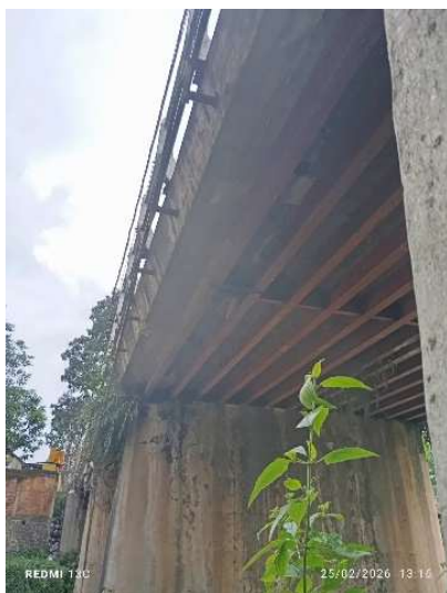
Figure 3 Corrosion on steel girder elements of Cikondang Bridge
