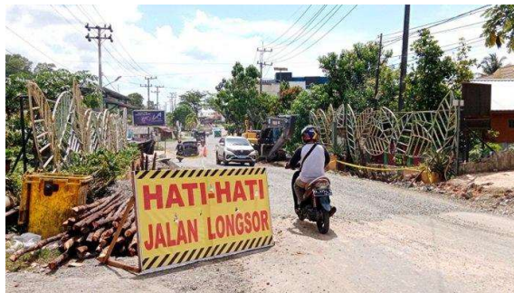
Figure 2 Temporary condition of the Sungai Salak Bridge
