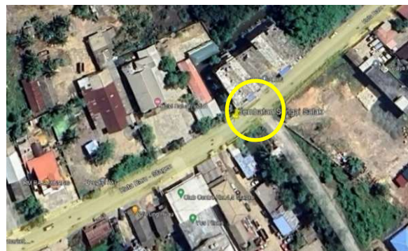
Figure 1 Location of the Sungai Salak Bridge assessment (Source: Google Earth, 2024)
